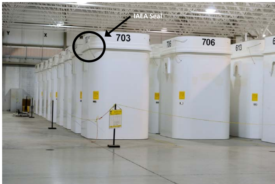
Figure 38: DSCs in Storage with IAEA Wire Seals
