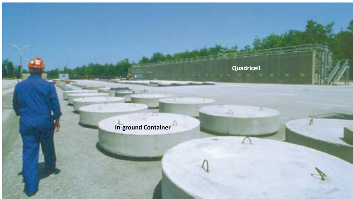
Figure 12: In-ground Containers (foreground) and Quadricells (background)
