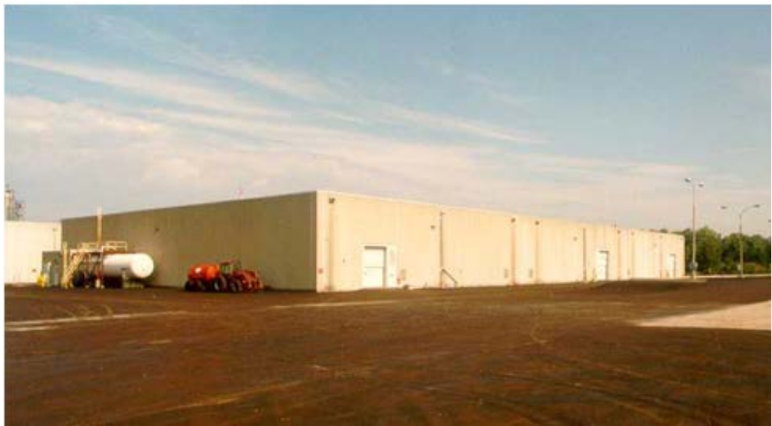
Figure 7: Low Level Storage Building
